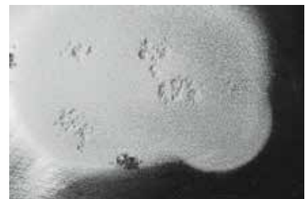
Rust pitting must be sand-blasted before the prepared area is ready for further treatment.
